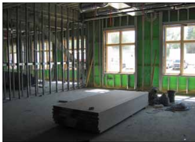
Spacious, well-lit classrooms are starting to take shape.
